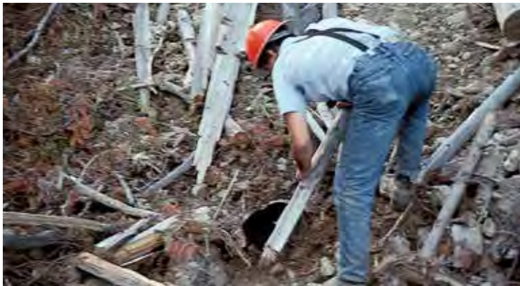
Hand, shovel, and chainsaw work are usually all that culvert maintenance requires. But don't delay! Delay in cleaning a blocked culvert or ditch can result in a damaged road that requires costly reconstruction.
