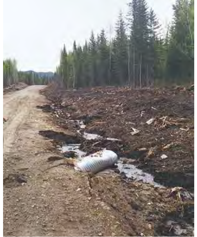
An unusually high flow event contributed to this blown out ditch which resulted in a relief culvert too high to drain under the road surface. A rock armored catch basin at the inlet could have reduced impacts on this site.
