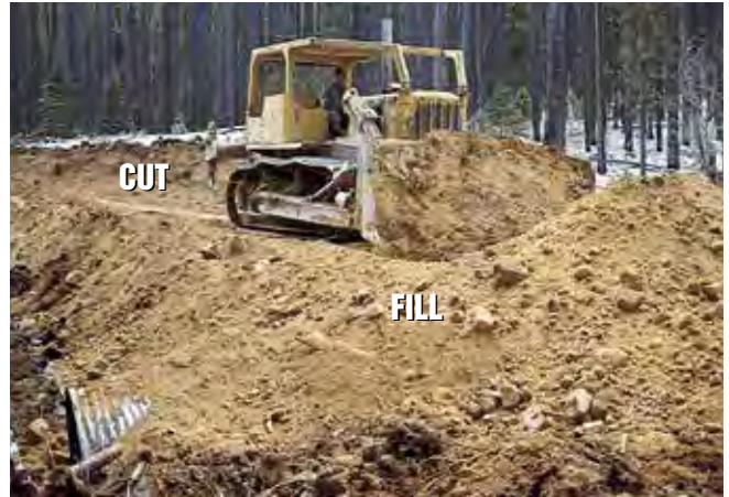
Cut-and-fill road construction is common for most terrain in Montana.
