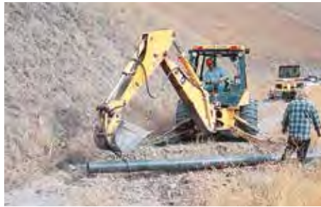
Skew pipe 30-45 degrees for self-cleaning. (15 foot roadbed requires 20 foot culvert)
