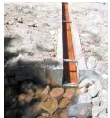
Open Top Wood Culvert
