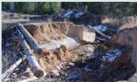
Ignoring BMPs can result in damaged streams, unhappy downstream neighbors, impassible roads, and fines.
