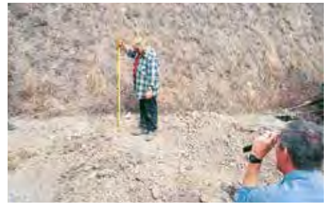
Pipe bed must have a grade of 8% to keep pipe working.
