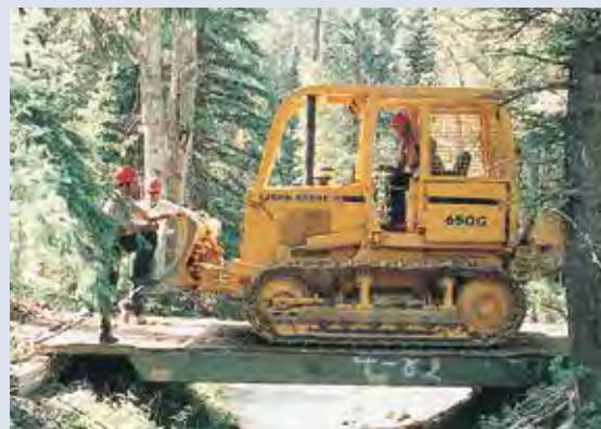
A portable bridge provides access across streams less than 10 feet wide with minimal disturbance to streambanks or bed (310 permit required). Select locations with firm soil banks, level grade, and minimal vegetation clearing.
