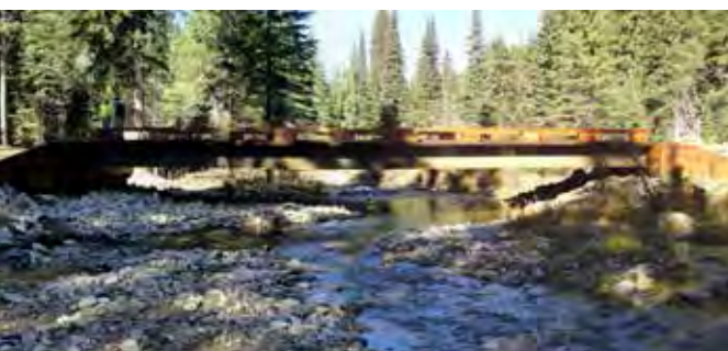
Bridges are best for large streams and those plagued with floatable debris problems. Bridges and arches have the least impact on fish.
