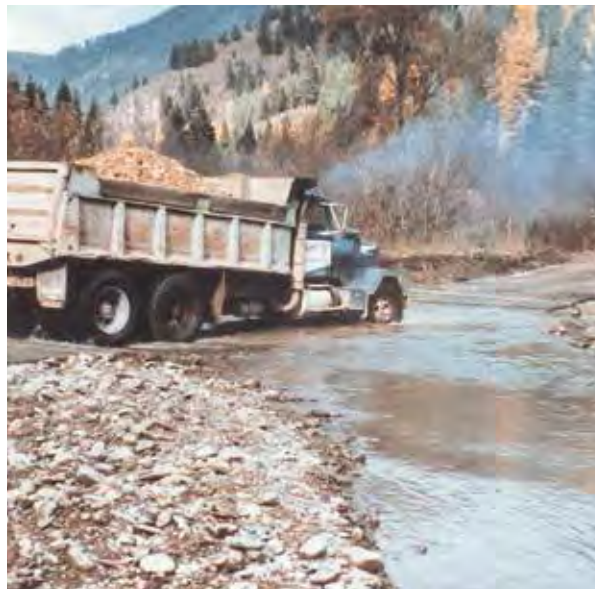
Limited traffic on this improved ford crossing has both minimal impact on the streambed and on sediment production.
