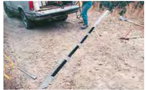
Slots are wide enough for cleaning but do not damage tires.
