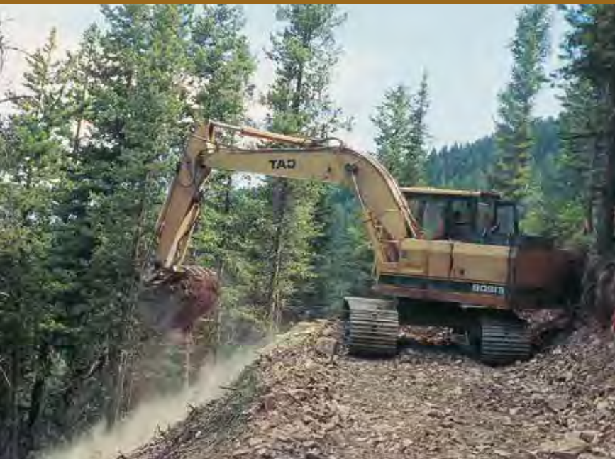
Excavator dismantling the road corridor.
