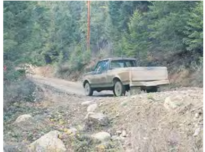
The drain dip bottom is sloped to carry water from the inside to the outside of a road surface and onto natural ground.
