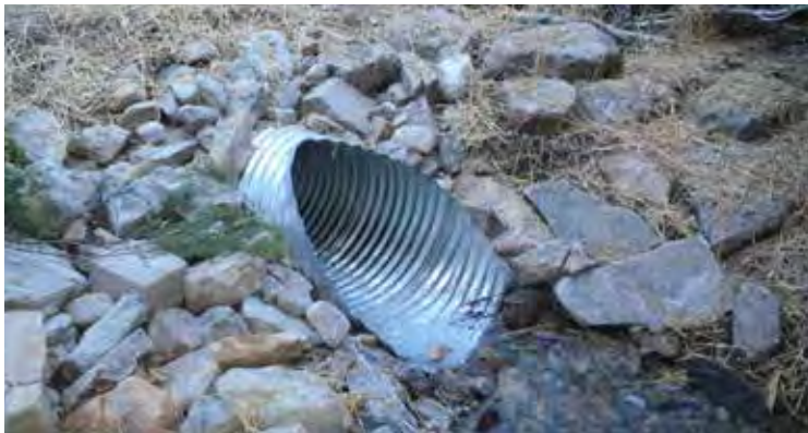
An armored culvert.
